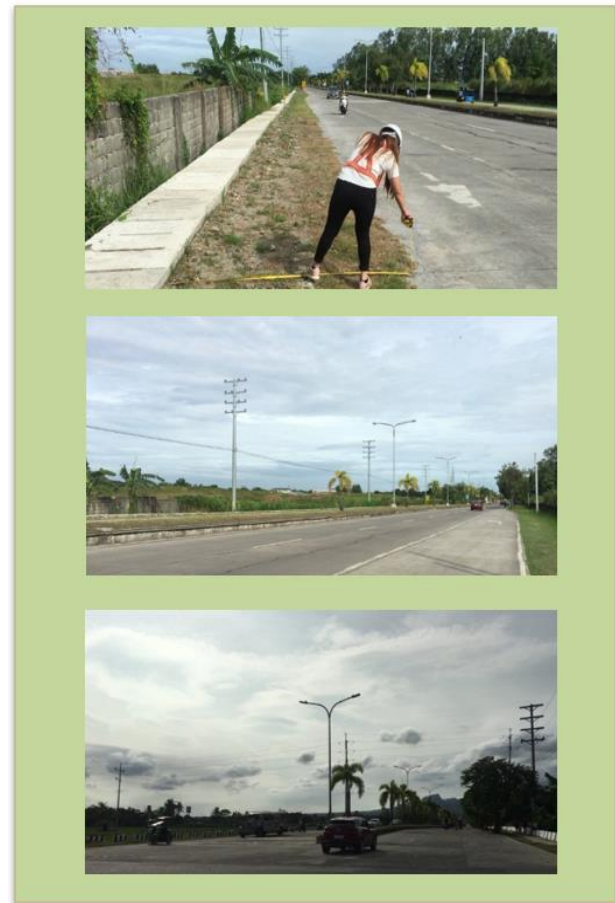
Fig.2. Existing Site Condition- Site Inspection/ Ocular Site Visit
