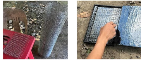
Fig.6. Installation of Wire Mesh
