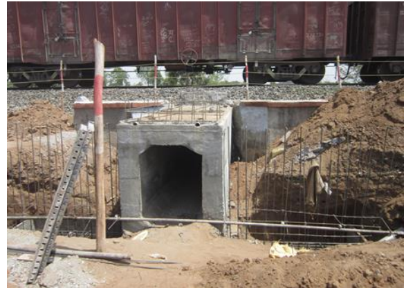
Fig.5. Br. No 863 in P-II Barrel portion completed
