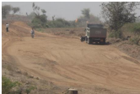
Fig.1. Earth Work Progress @ Km 625.100
