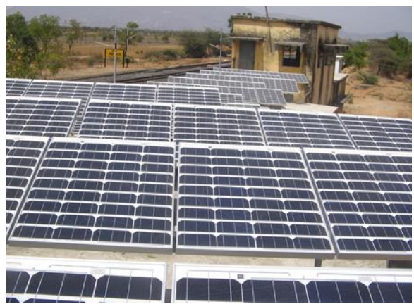
Fig.7. Solar Panel Erected at Jetti Station In P-II
