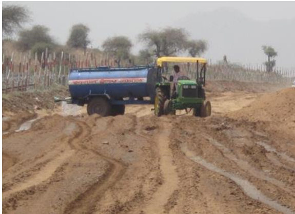
Fig.2. Embankment Progress @ Km 625
