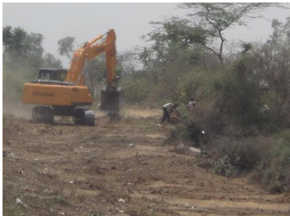
Fig.3. CNG Progress @ Km 625.5
