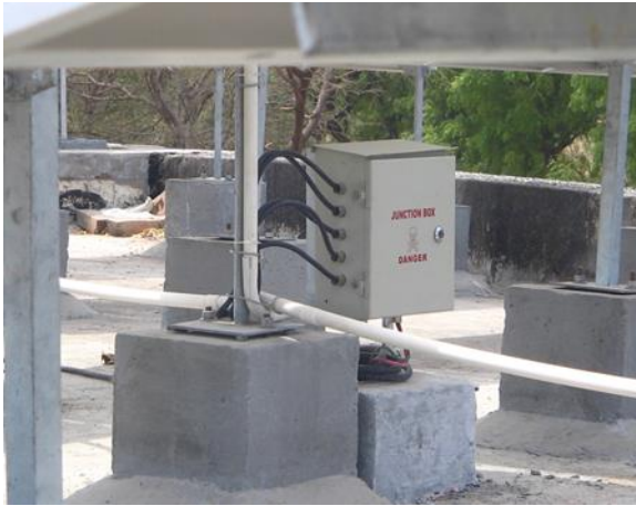
Fig.8. Solar Module Erected at Korjoda Station
