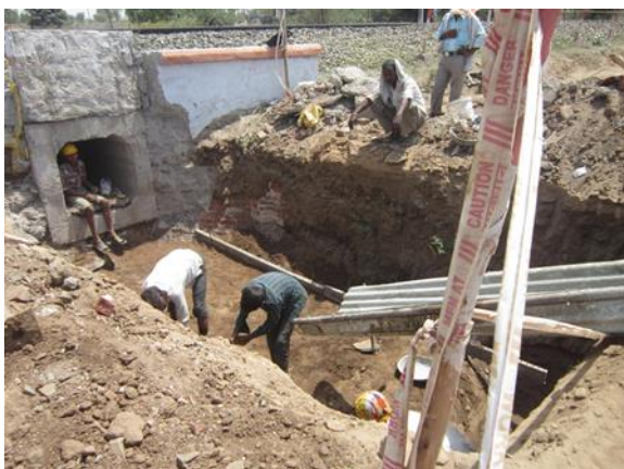
Fig.4. Br. No 862 PCC Progress
