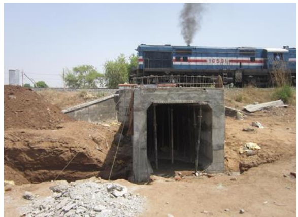
Fig.6. Br. No 864 in P-II Barrel Portion Completed
