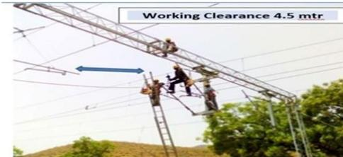
Fig.6. Cantilever adjustment
