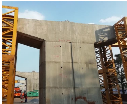
Fig.6. Complex structure of pier
