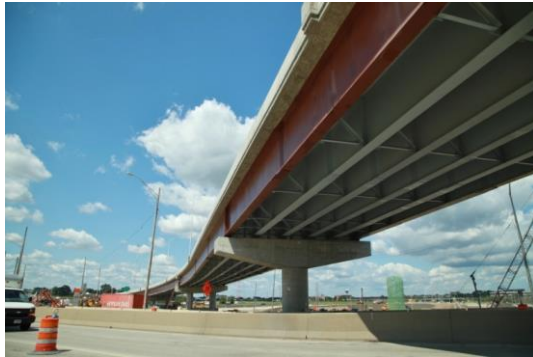
Fig.7. Structural element of the superstructure of a bridge
