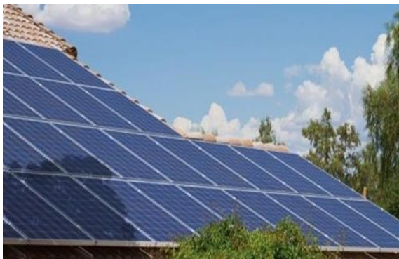
Fig.1. Partial shading of PV module
