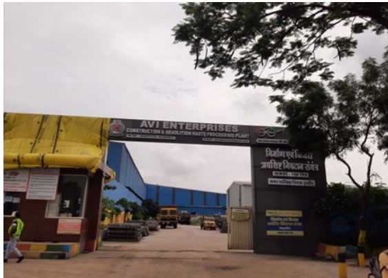
Fig.2. C&D Waste recycling plant in Indore, India.
