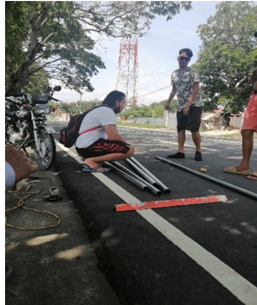
Fig.5. Constructing the poles that will use to hold the streetlight
