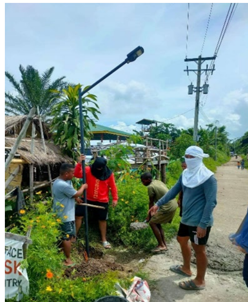
Fig.6. Installation of the streetlight
