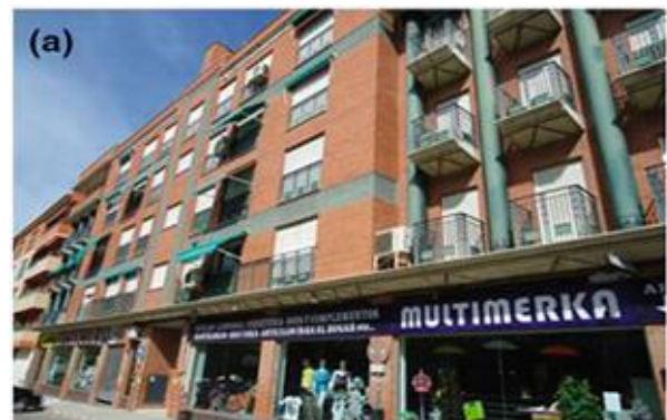
Fig.7(a). Building with soft storey
