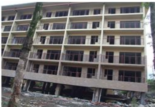
Fig.4. Formation of weak storey: leaned 6-story building in Dujiangyan
