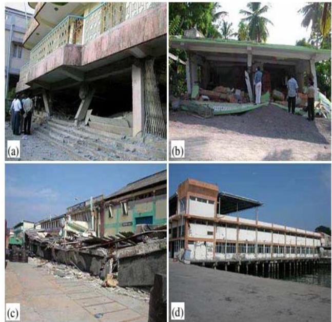
Fig.2. Collapse of RC buildings at (a) Naya Gaon, (b) Bamboo Flat, and (c) Haddo wharf, and (d) partially collapsed Passenger Terminal Building at Haddo wharf.
