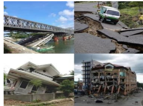
Fig.3. Damage done by Earthquake to Horizontal and Vertical Structures
