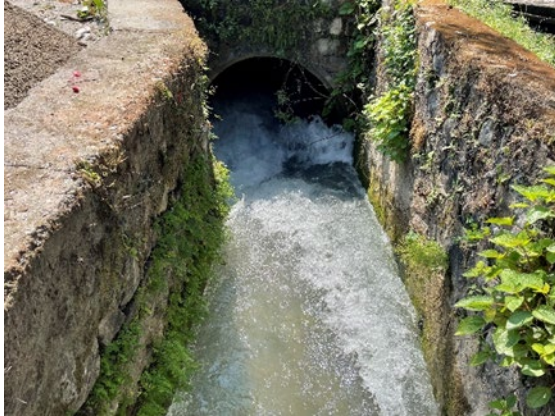
Fig.4 on-site water channel.
